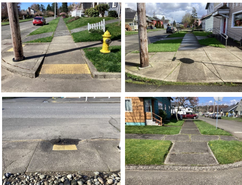
Top left: Non-compliant Grade A ramp. Top right: Non-compliant Grade B ramp. Bottom left: Non-compliant Grade C ramp. Bottom right: Non-compliant Grade D missing ramp.
