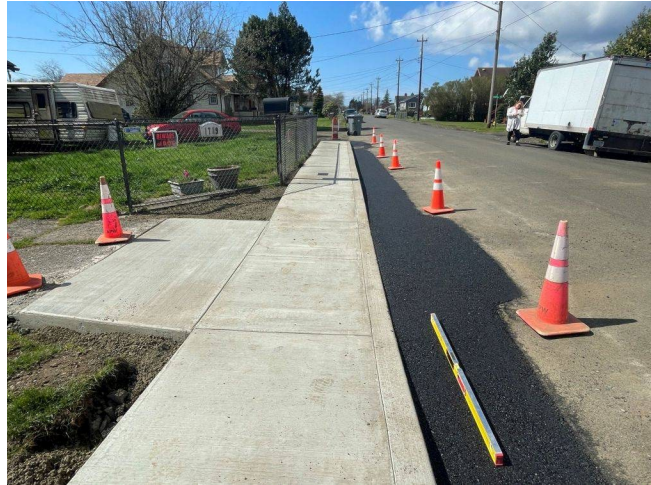
Photo of a compliant driveway and sidewalk interface with required width, running slope, and cross slope on Morgan St in the City of Aberdeen.
