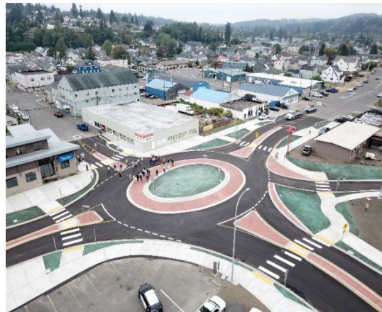
New ADA-compliant curb ramps, sidewalk, and driveways at F Street/Market Street roundabout.
