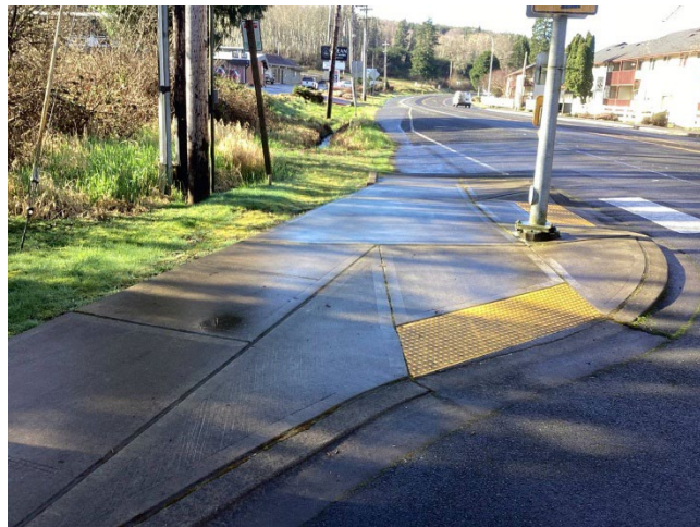
Photo of compliant curb ramp with required width, running slope, cross slope, and detectable warning surface (DWS) on SE corner of SR 105 and Edward P. Smith Drive.
