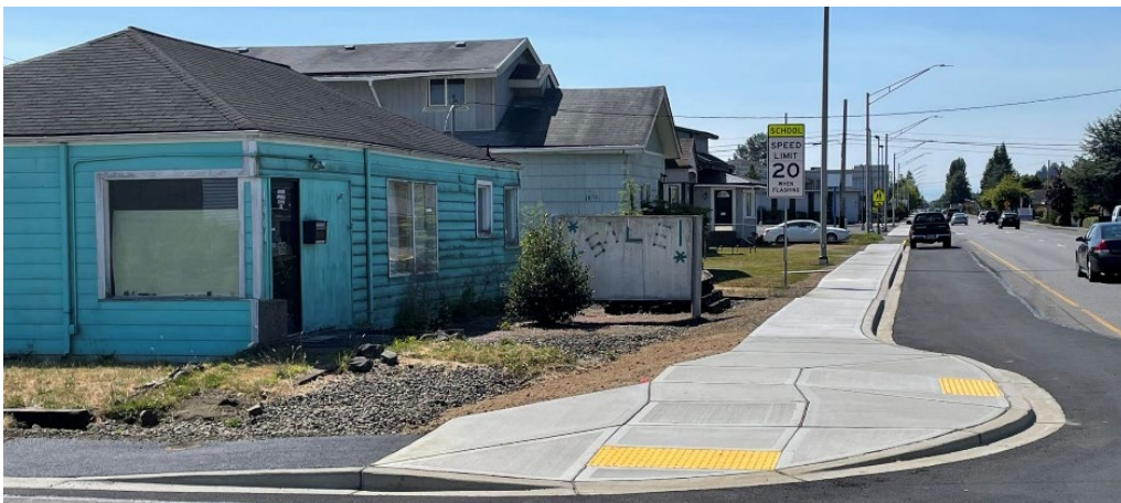
New ADA-compliant curb ramps, sidewalk, and driveways on south side of westbound US 12 west of Jeffries St.
