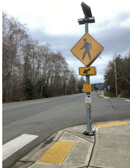
Photo of compliant RRFB pushbutton on east side of SR 105 at Edward P Smith Drive that meets ADA requirements for reach and clear space and PROWAG features.
