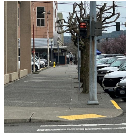
Photo of non-compliant pedestrian signal that lacks audible locator tone and crossing notification on southeast corner of Broadway St and Market St.
