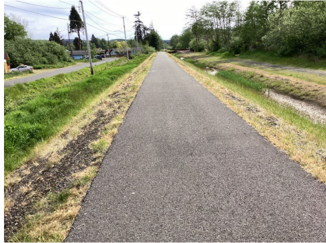
Photo of a compliant section of the Chehalis Riverfront Walkway that meets ADA requirements for width, running slope, and cross slope.
