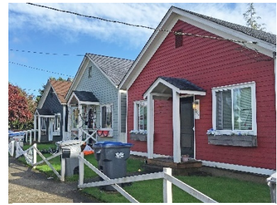
Figure 3-8. Compact traditional residential architecture. Source: MAKERS
