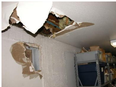
Evidence room – still leaking after several repairs
